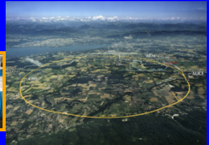
Damage at the LHC 2008 / 09 / 19
